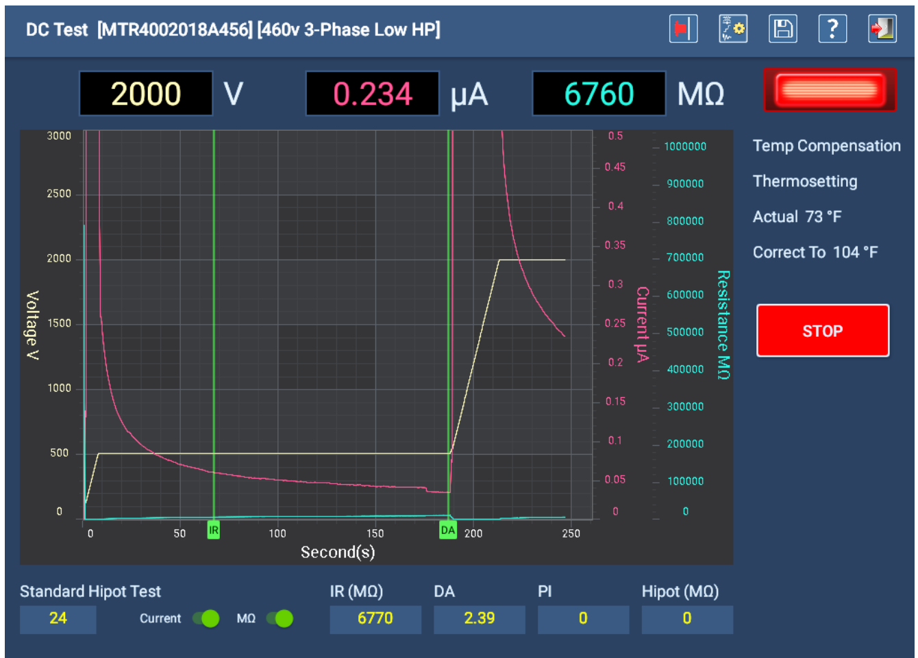
Fig 124: Auto DC Test screen—test in progress.
